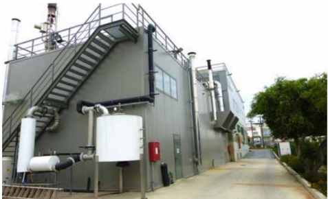
The Heraklion Biogas Plant features here in this part of the facility a special deodorization system that enables plant's integration into the urban environment and a highly specialized wastewater treatment system for the effluents avoiding any contamination of the environment.
